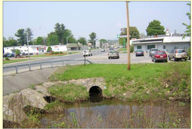
A new underground stormwater treatment structure will capture runoff from Route 9 and the surrounding developed area. The structure will be installed in the lawn area above, on Enterprise Rent-a-Car property.
